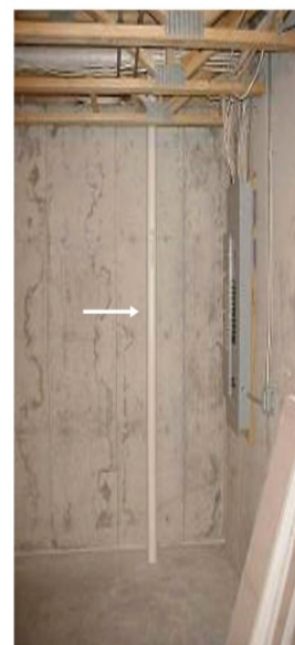
Photo: A vapor control system installed in the basement of a house.
