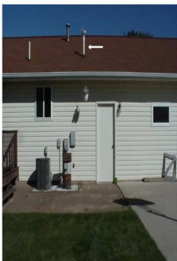
Photo: A Study Area house with a vapor control system where the pipe vents through the roof at the back of the house. The vapor control system pipe is the farthest right, and has a small wind turbine at the top. This is one option for extending the pipe outside of a structure and above the roof line.
